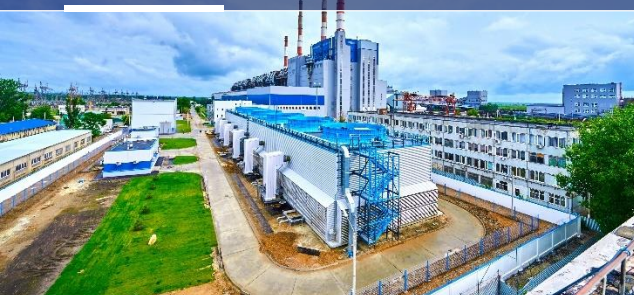
Construction of the 9 th power block of the Novocherkassk power station ▶
